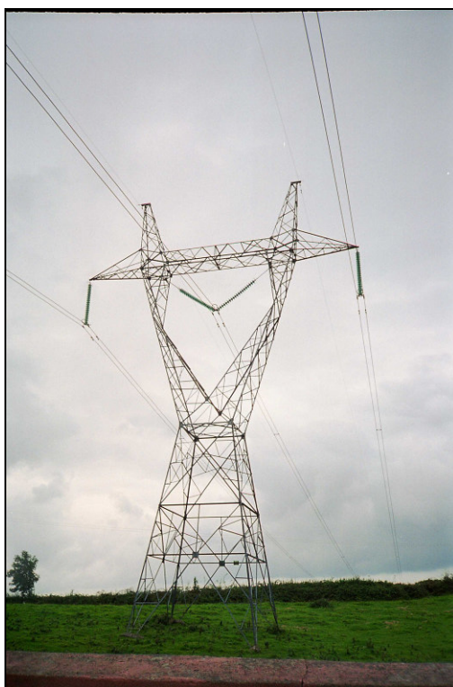
Figure 3.1 Typical 400kV Overhead Line Structure
